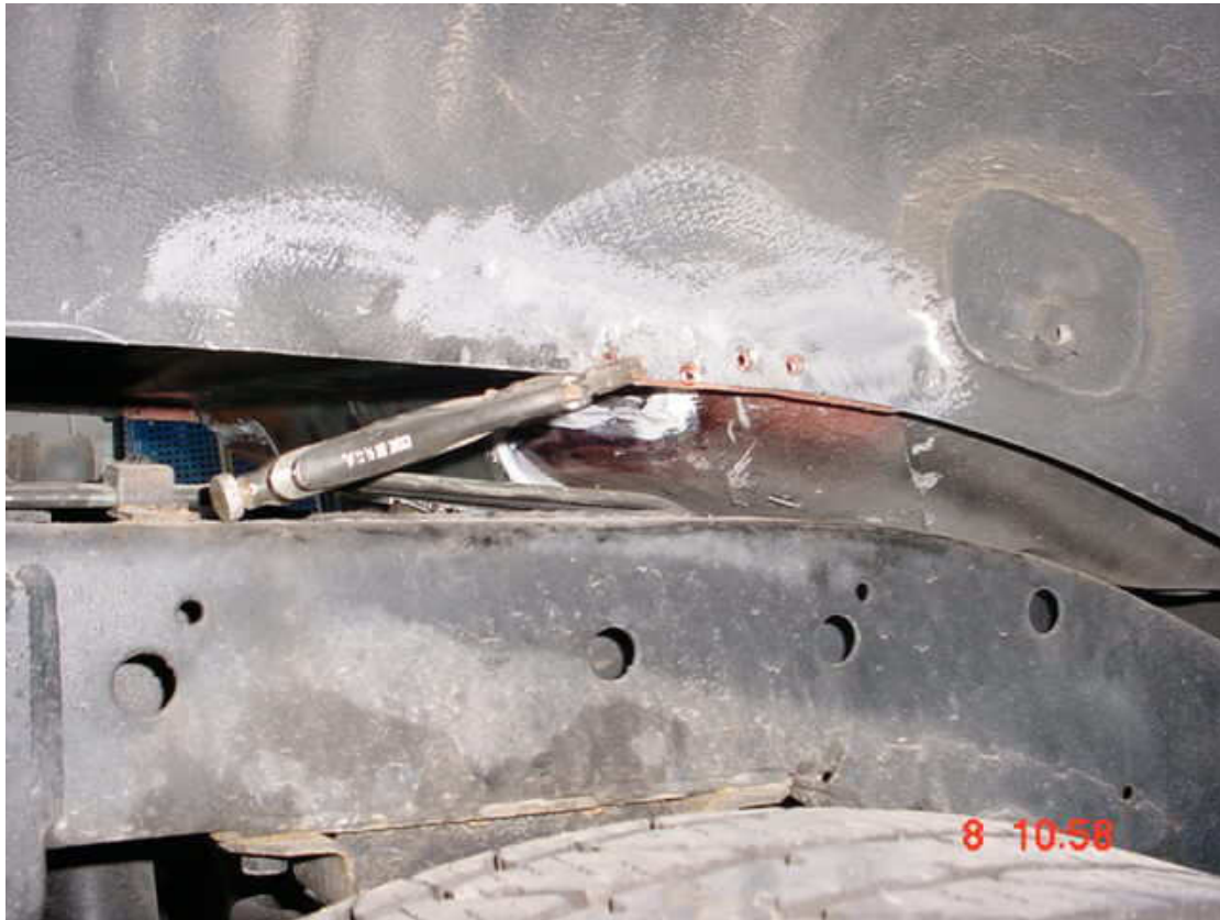
Plug-welds in wheel-arch area are about to be welded.
