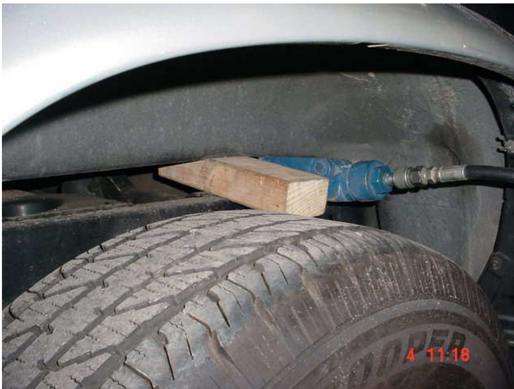
The body is lifted away from the rear end of the chassis and supported by approximately 100mm solid blocks.
