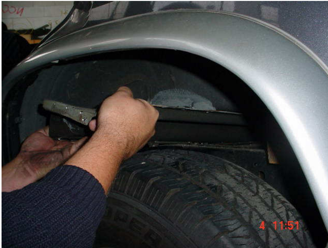
The reinforcing plate is manoevered out through the gap between the wheel-arch and the chassis rails.
