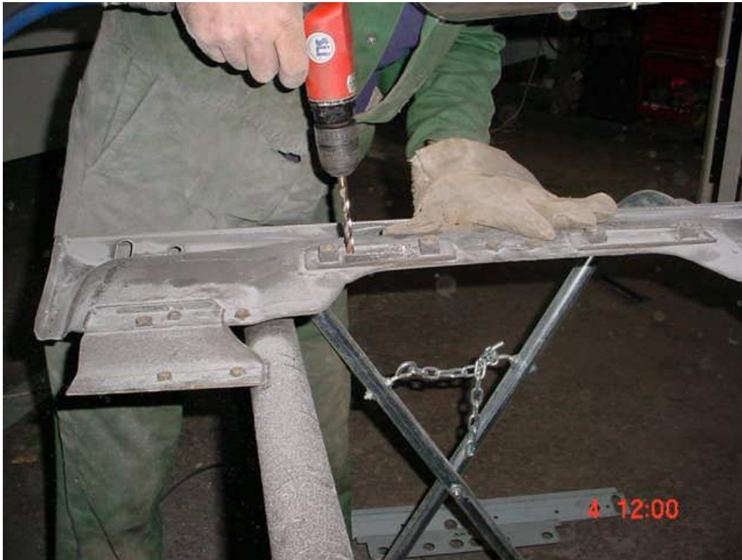
The spot welds holding the seat-belt anchorages to the reinforcing plate are drilled through 2mm (both layers) then 8.5 mm through the anchorage plate only (1 layer).
