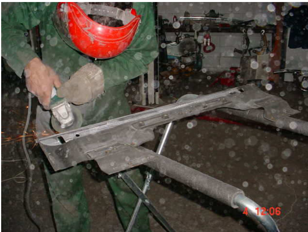
The reinforcing plate underside is cleaned to bare metal by wire-wheel and grinding to remove rust, etc and where the LVV load-bar overlaps.
