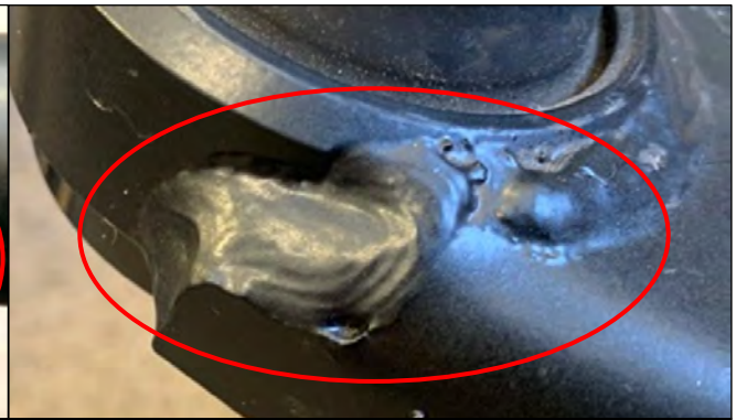
Image 4: This is an example of a poor weld including craters and incomplete welds at the ball joint end housing.
